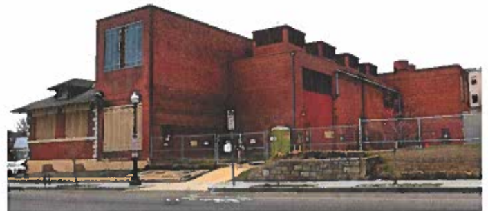
Current Harvard Substation
